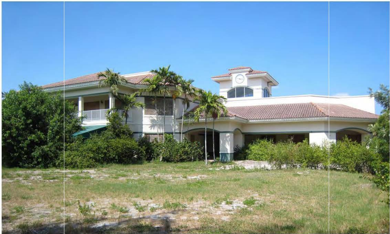
View of Existing Club House
