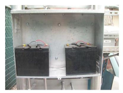
Figure 3: Battery Compartment
