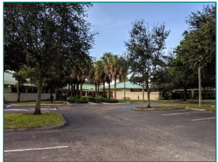
1 Front of shelter
