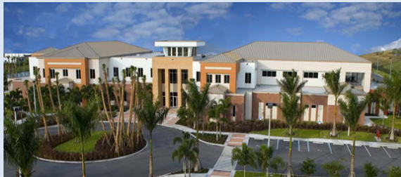
Fire Rescue Headquarters
