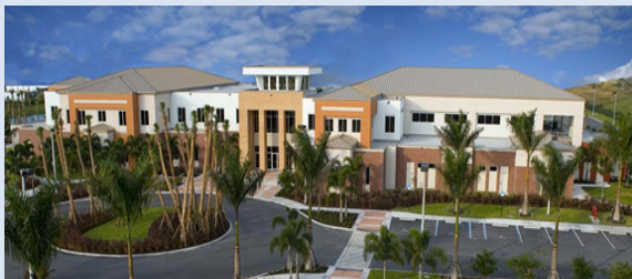
Fire Rescue Headquarters
