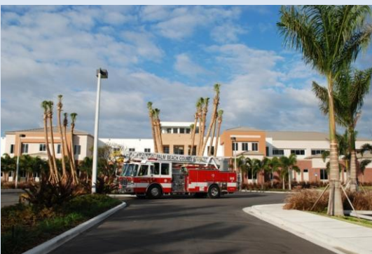
Fire Rescue Headquarters
