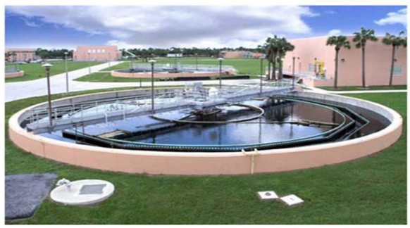
Southern Regional Water Reclamation Facility
