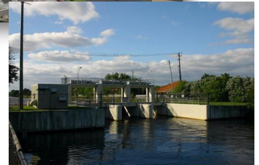
G-54 Structure (Sewell Lock) and flooding in Ft Lauderdale 2020.
