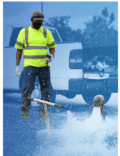
Conducting pipeline flushing
