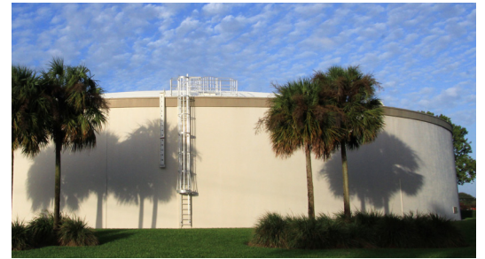
Water Storage Tank at Water Treatment Plant 3
