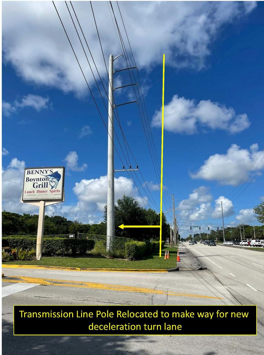
Transmission Line Pole Relocated to make way for new deceleration turn lane
