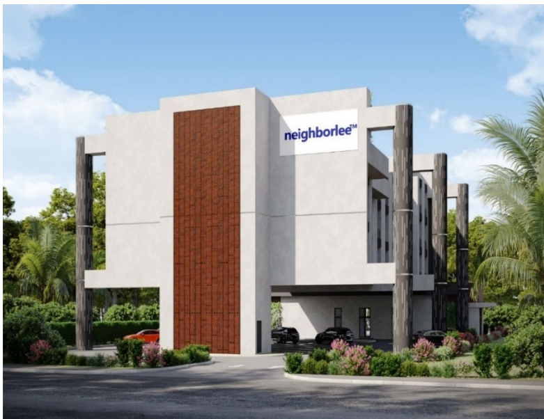
Figure 9. South Elevation, view from Nokomis Ave.
