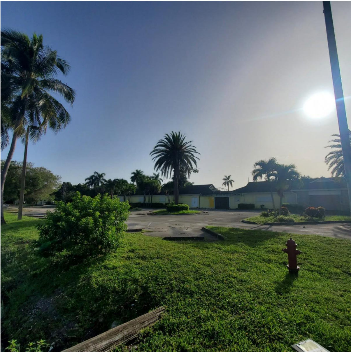
View of vacant Cypress Creek Golf Course Clubhouse and parking lot. Camera view Northeast.
