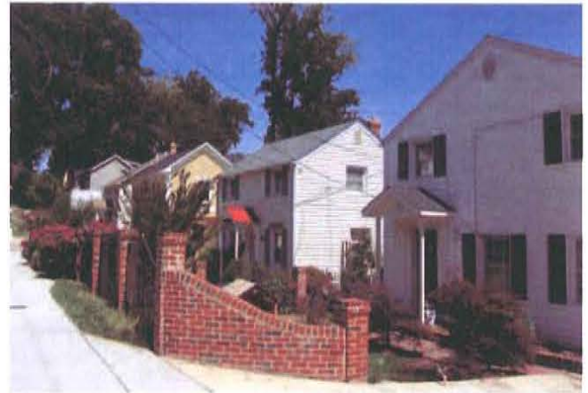
Figure 45. Claremont Historic District in Arlington County, Virginia. Although some of the homes have replacement siding and windows, as a collection, the district is able to convey significance as a planned neighborhood of affordable housing (Mead & Hunt photograph).
