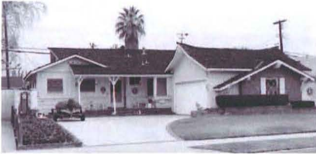
Figure 31. Storybook style house in Los Angeles, California, constructed c.1958, retains its massing and materials and displays multiple architectural elements, including sweeping gables, scalloped bargeboards, and diamond-pane windows. As a result, it meets the survey criteria (Mead & Hunt photograph).
