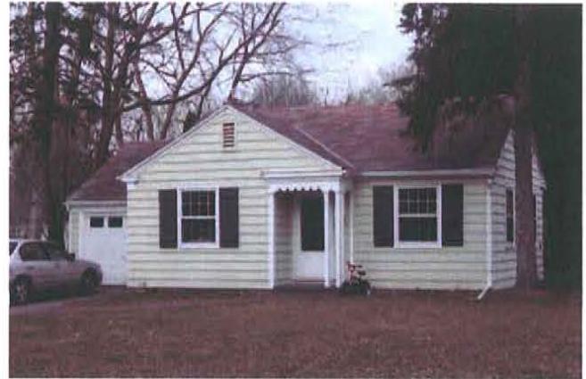
Figure 112. Minimal Traditional house in Madison, Wisconsin, constructed c.1945, with wood siding, compact one-story plan, minimal eave overhang, inset entrance, attached one-car garage, and modest Colonial Revival details, including gable end returns and cornice boards (Mead & Hunt photograph).
