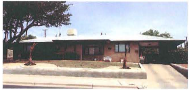
Figure 128. Ranch house in El Paso, Texas, constructed c.1960, with horizontal massing, hip roof, picture windows, glass block windows at the entrance, minimal wrought iron details, and carport (Mead & Hunt photograph).
