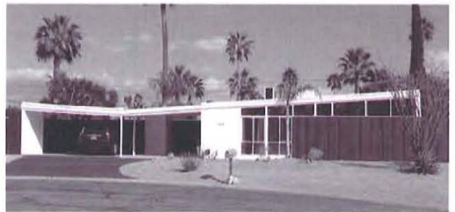
Figure 155. Contemporary style house in Palm Springs, California, constructed c.1954, with low-pitched roof, glass curtain wall, de-emphasized entrance, and attached carport (photograph courtesy of Andrew Hope, Caltrans).
