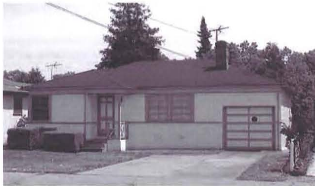
Figure 121. Transitional Ranch in San Lorenzo, California, with compact massing, integrated garage, and recessed entrance. The house was constructed by merchant builder Dave Bohannon c.1950 (photograph courtesy of Andrew Hope, Caltrans).
