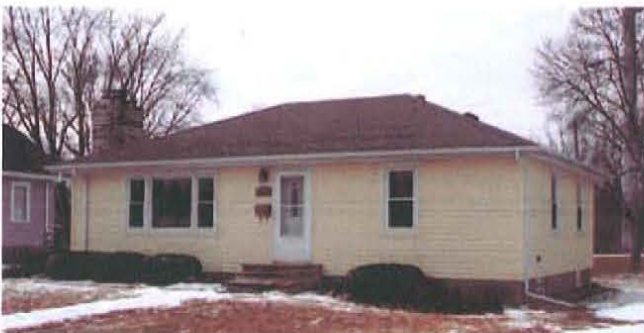
Figure 14. Transitional Ranch house in St. Louis Park, Minnesota, constructed in 1953, does not meet the survey criteria due to the replacement vinyl siding and windows (Mead & Hunt photograph).
