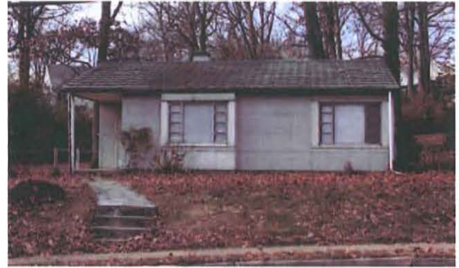
Figure 162. Lustron house in Arlington County, Virginia, erected in 1949, retains the porcelain enamel dove gray siding, steel roof, inset entry and support post, and steel windows (Mead & Hunt photograph).
