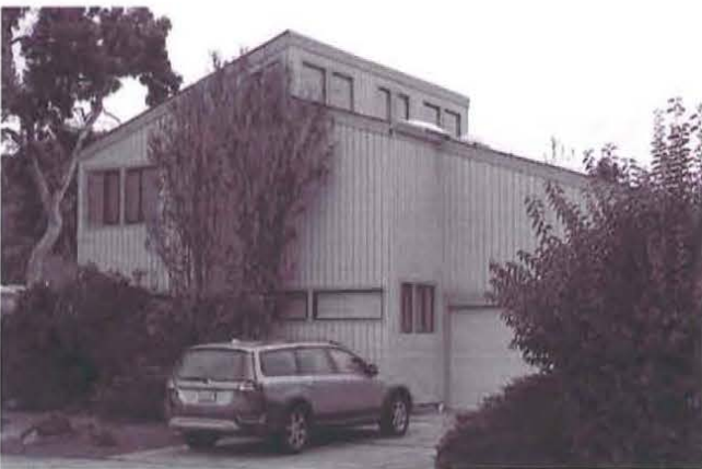
Figure 157. Shed house in Palo Alto, California, constructed c.1972, with intersecting shed roof lines, wood siding, clerestory windows, and an integrated garage (photograph courtesy of Andrew Hope, Caltrans).
