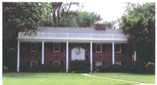
Figure 30. Georgian Revival house in Fairfax County, Virginia, retains the original materials and massing; displays multiple architectural elements, including a colonnaded portico, quoins, and door surround. As a result, it meets the survey criteria (photograph courtesy of Anne Bruder, Maryland State Highway Administration).
