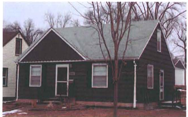
Figure 2. Intact c.1945 house in the postwar St. Louis Park, Minnesota, neighborhood. This residence represents the Minimal Traditional form with a side gable roof and prominent gable above the entrance. The house retains the original footprint, wood shingle siding, and double-hung windows (Mead & Hunt photograph).
