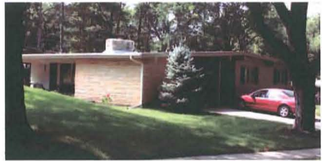
Figure 172. Patio located at rear elevation of c.1956 Ranch house in Lincoln, Nebraska (Mead & Hunt photograph).
