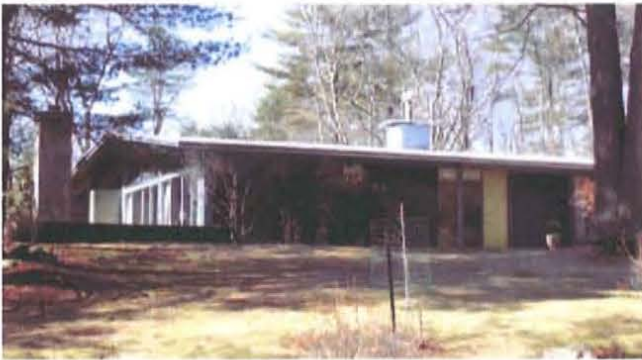
Figure 93. Detail of ALCOA Care-free House in Lincoln, Massachusetts (photograph courtesy of John A. Burns, FAIA).
