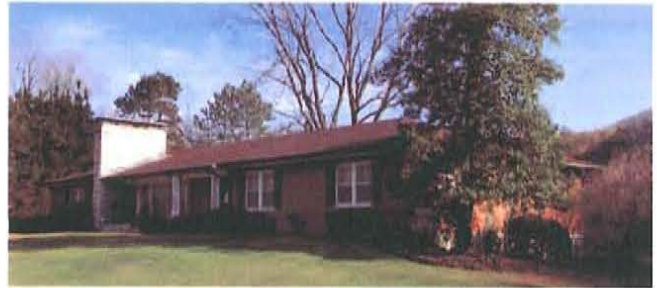
Figure 129. Ranch house in Richmond Heights, Missouri, with horizontal massing, hip roof, integrated stone planters, prominent stone chimney, and wrought iron supports at the entrance (photograph courtesy of Toni Prawl, Missouri Department of Transportation).
