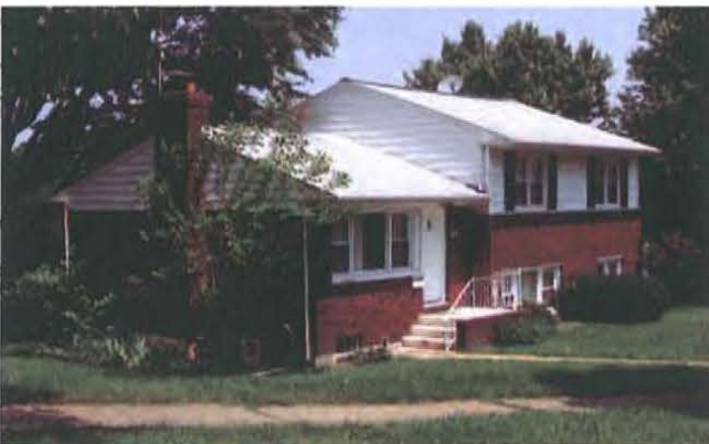
Figure 138. Split-level house in Baltimore County, Maryland, with an elevated entry, brick veneer, and picture window (photograph courtesy of Anne Bruder, Maryland State Highway Administration).
