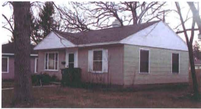
Figure 168. Harnischfeger prefabricated home in Madison, Wisconsin, erected c.1950 (Mead & Hunt photograph).
