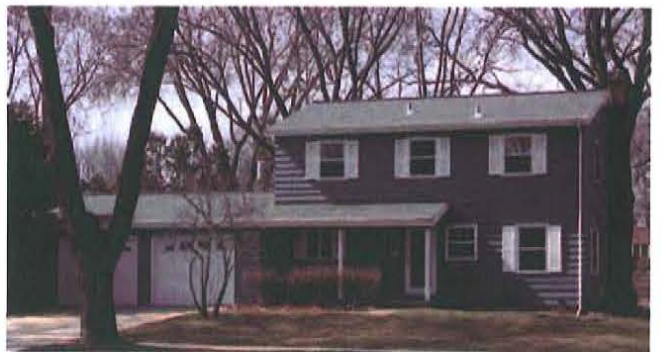
Figure 120. Two-story Massed house in Madison, Wisconsin, constructed in 1959, featuring a rectangular plan, two-story massing, and side gable roof (Mead & Hunt photograph).
