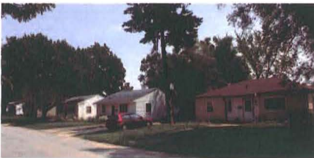
Figure 73. Collection of c.1950 Minimal Traditional and Transitional Ranch homes in Madison, Wisconsin, with substantial alterations to the majority of properties, including non-compatible siding, replacement windows, and altered entrances and carports (Mead & Hunt photograph).
