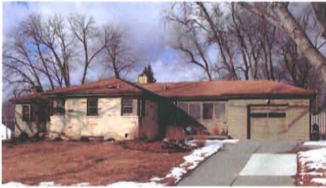
Figure 125. Ranch house in Omaha, Nebraska, constructed c.1955, with horizontal massing, hip roof, clapboard and stone veneer, picture and double-hung windows, and attached breezeway and garage (Mead & Hunt photograph).
