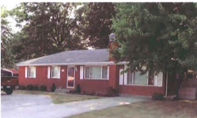
Figure 18. Ranch house in Grain Valley, Missouri, does not meet the survey criteria due to absence of architectural elements and altered attached garage that has been converted into living space (photograph courtesy of Toni Prawl, Missouri Department of Transportation).
