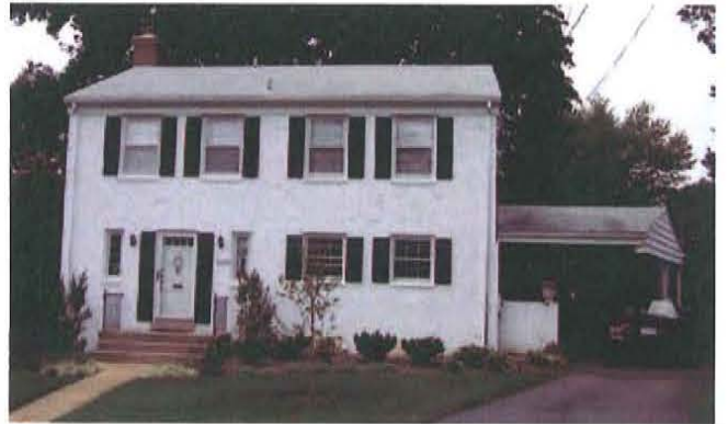
Figure 119. Two-story Massed house in Arlington County, Virginia, featuring a rectangular plan, two-story massing, and side gable roof (Mead & Hunt photograph).
