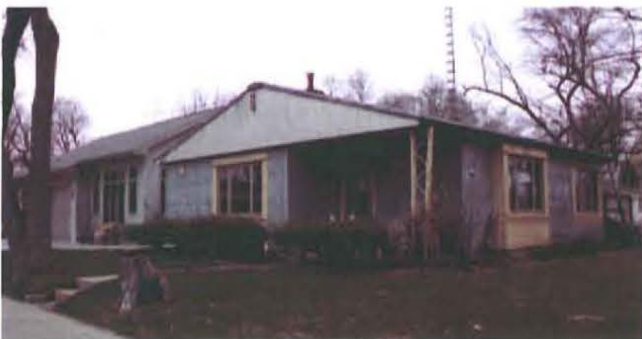
Figure 39. Although this c.1950 Lustron house in Oshkosh, Wisconsin, has replacement casement windows and a large modern addition, it should be surveyed due to the limited number of Lustrons constructed nationwide (Mead & Hunt photograph).
