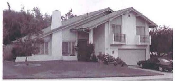
Figure 150. Spanish Colonial Revival style applied to the Split-level form in La Mesa, California, constructed c.1970, with stucco exterior and tile roof (photograph courtesy of Andrew Hope, Caltrans).
