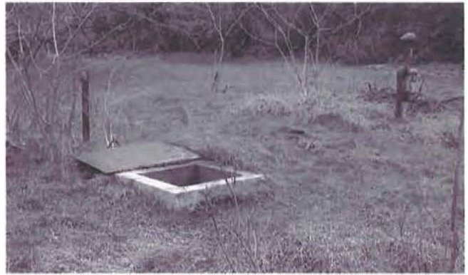
Figure 176. Bomb shelter in Sonora, California, constructed c.1960, from left to right are the exhaust air vent, hatch, and fresh air intake (photograph courtesy of Andrew Hope, Caltrans).
