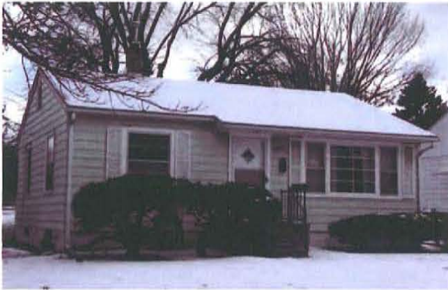
Figure 9. Minimal Traditional house in Omaha, Nebraska, constructed c.1945, retains its original siding, massing, simple entrance, and windows, and thus meets the survey criteria (Mead & Hunt photograph).
