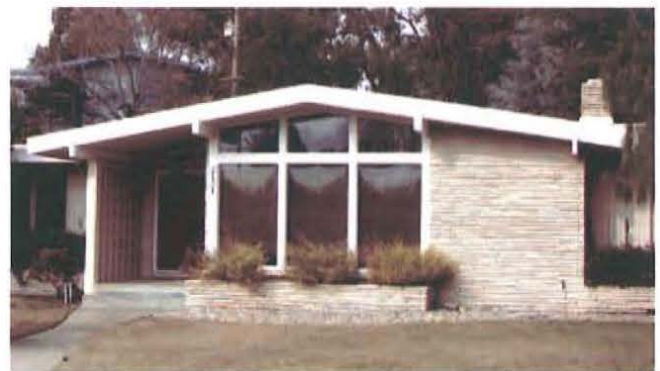
Figure 97. Concrete screen at the front entrance of a c.1964 Ranch house in Sacramento, California (photograph courtesy of Andrew Hope, Caltrans).
