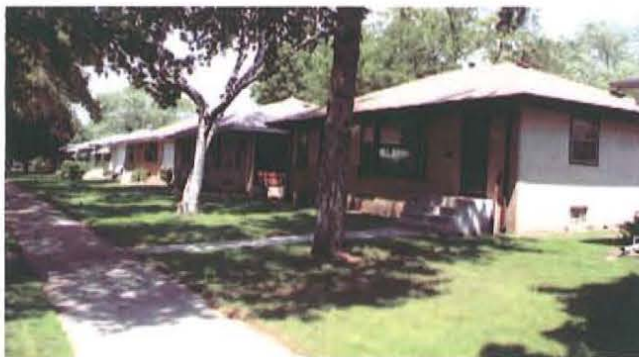
Figure 123. Transitional Ranch homes in Minneapolis, Minnesota, constructed c.1950, exhibiting horizontal massing, compact floor plans, and picture windows and accent veneer on the facades (Mead & Hunt photograph).
