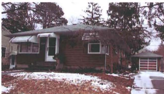
Figure 122. Transitional Ranch in St. Louis Park, Minnesota, constructed c.1950, with compact massing, corner windows, low-pitched roof with a wide eave overhang, and attached garage at the rear (Mead & Hunt photograph).
