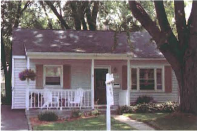
Figure 38. Prefabricated National Homes residence in Madison, Wisconsin, constructed c.1951, retains its massing and roofline, but is clad in non-compatible narrow-gauge vinyl siding. As a result, it does not meet the survey criteria (Mead & Hunt photograph).
