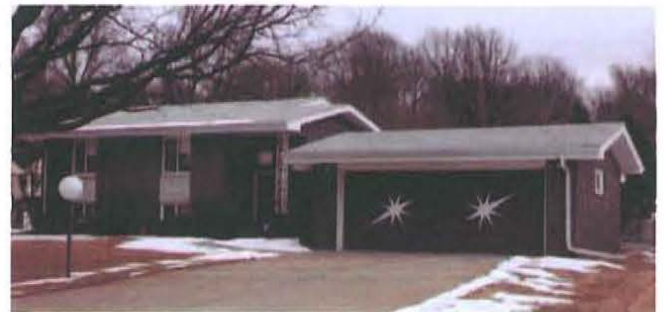
Figure 23. Split-level residence in Omaha, Nebraska, constructed c. 1965, retains its original form, doors and windows, and displays multiple architectural elements, including accent stone veneer, wrought iron support, and prominent front entrance. As a result, it meets the survey criteria (Mead & Hunt photograph).
