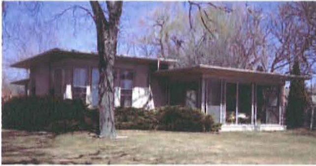
Figure 67. Contemporary house in Oshkosh, Wisconsin, constructed c.1960, with cumulative alterations, including vinyl siding, and an altered patio; it is not considered individually eligible under Criterion C: Architecture (Mead & Hunt photograph).
