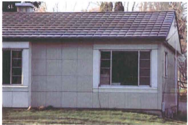
Figure 95. Porcelain enamel coated steel panels on a c.1950 Madison, Wisconsin, Lustron home (Mead & Hunt photograph).
