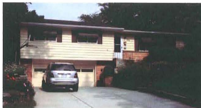
Figure 131. Raised Ranch in Madison, Wisconsin, constructed c.1960, with a partially exposed basement, integrated garage, picture window, overhanging eaves, wide chimney, and accent brick veneer (Mead & Hunt photograph).
