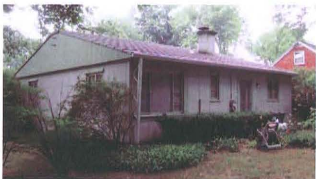
Figure 164. Rear elevation of a Lustron house in Glenville, New York, erected in 1949, that retains the porcelain enamel dove gray siding, steel roof, support post, and steel windows (photograph courtesy of Kimberly Konrad Alvarez, Landmark Consulting LLC/NYS Lustron Project Coordinator).
