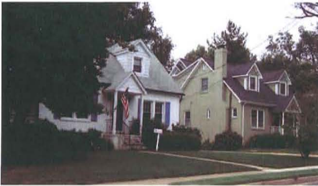
Figure 116. Cape Cod houses in Arlington County, Virginia, constructed c.1950, with one-and-one-half-story massing, symmetrical facades, central entrances with pedimented stoops, and steeply pitched side gable roofs with dormers and double-hung windows (Mead & Hunt photograph).
