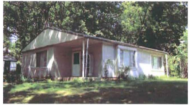
Figure 17. A Lustron house erected in 1949 at 1124 South Forest Drive in Virginia Heights (Mead & Hunt photograph).
