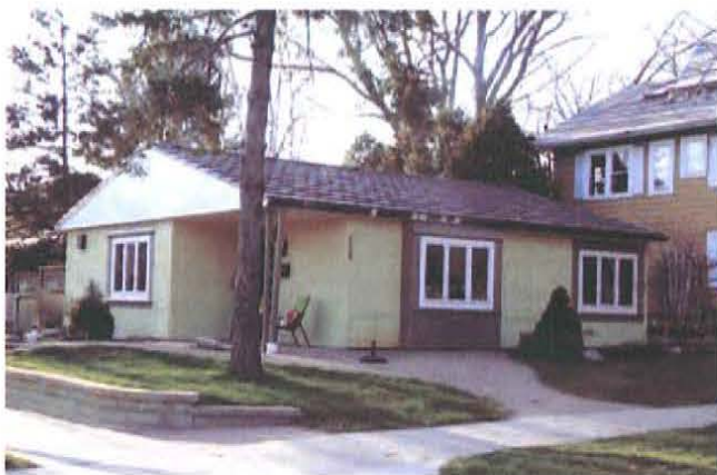
Figure 163. Lustron house in Madison, Wisconsin, erected c.1950, retains the porcelain enamel maize yellow siding, steel roof, and inset entry and support post; the windows have been replaced (Mead & Hunt photograph).
