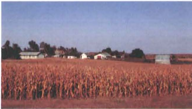
Figure 77. Postwar c.1960 Ranch house added to an early twentieth-century farmstead in rural Dawson County, Nebraska (Mead & Hunt photograph).
