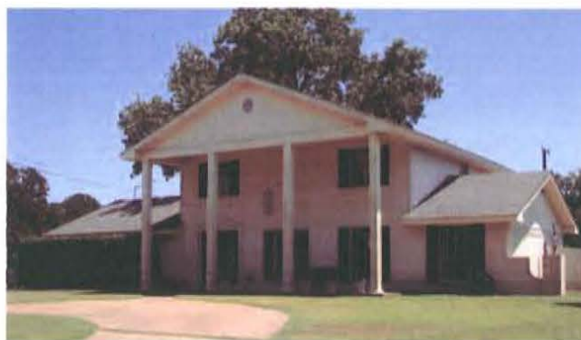
Figure 27. Colonial Revival in Arlington, Texas, constructed in 1967, retains its original materials and massing and displays multiple architectural elements, including a decorative door surround, projecting front gable, and compass vent. As a result, it meets the survey criteria (Mead & Hunt photograph).
