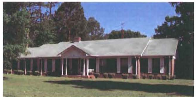
Figure 144. Ranch house in Fort Valley, Georgia, constructed c.1960, with Colonial Revival architectural details, including multi-light windows with faux shutters and an entrance stoop with decorative columns and dentils (photograph courtesy of Georgia Department of Natural Resources, Historic Preservation Division).
