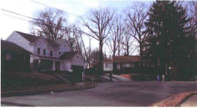
Figure 72. Large infill house under construction in Arlington County, Virginia, that detracts from the size and scale of the 1950s Transitional Ranch neighborhood (Mead & Hunt photograph).
