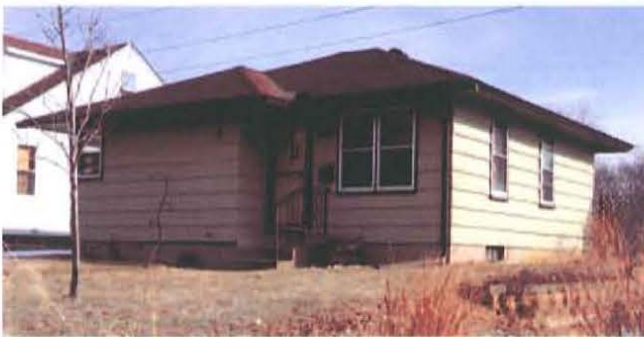
Figure 4. Intact c.1950 house in the postwar St. Louis Park, Minnesota, neighborhood. This residence represents the Transitional Ranch form. The house retains the original footprint, wide-lap wood siding, and double-hung windows, which are partially obscured by modern storm windows (Mead & Hunt photograph).
