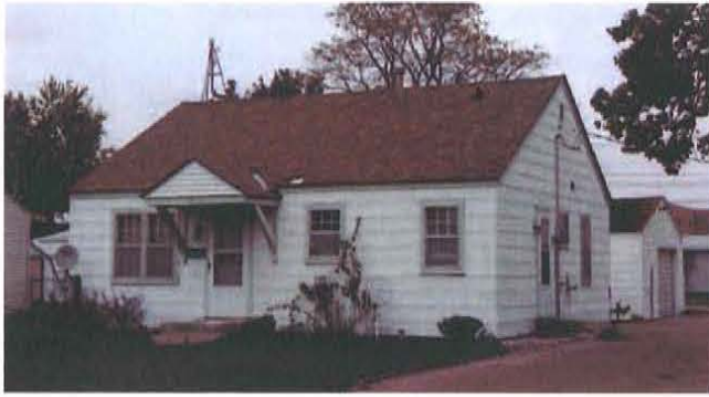
Figure 113. Minimal Traditional house in Gothenburg, Nebraska, constructed c.1945, with a compact one-story plan, asbestos shingle siding, double-hung windows, and simple portico (Mead & Hunt photograph).
