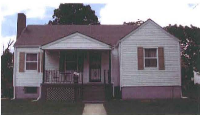
Figure 10. Minimal Traditional house in Prince George's County, Maryland, constructed c.1945, with non-compatible vinyl siding, replacement windows, and a modified stoop. As a result, it does not meet the survey criteria (photograph courtesy of Anne Bruder, Maryland State Highway Administration).
