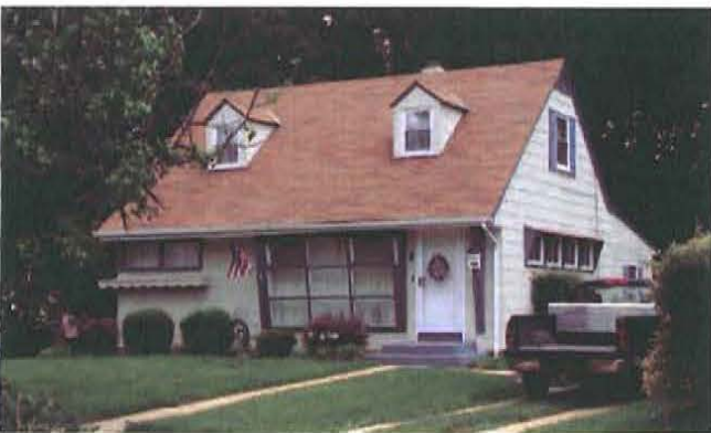
Figure 117. Cape Cod house in Fairfax County, Virginia, with one-and-one-half-story massing, side gable roof with twin dormers, and canted front picture window (photograph courtesy of Anne Bruder, Maryland State Highway Administration).
