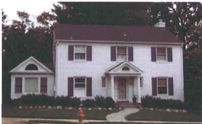
Figure 29. Colonial Revival house in Arlington County, Virginia, has an altered front portico and modern side addition. As a result, it does not meet the survey criteria due to lack of historic integrity (Louis Berger photograph).
