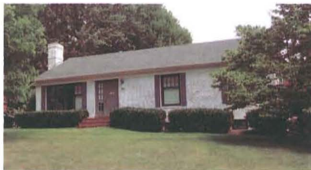
Figure 20. Ranch house in Arlington County, Virginia, constructed in 1959 that does not meet the survey criteria because the multi-light, “cottage-style” replacement windows are non-compatible. In addition, it does not display three architectural elements (Louis Berger photograph).
