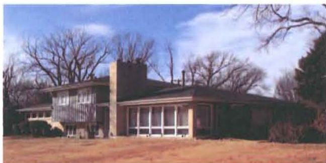
Figure 24. Split-level residence in Richmond Heights, Missouri, retains its original form, and displays multiple architectural elements, including accent board and batten siding, prominent chimney, and bands of windows. As a result, it meets the survey criteria (photograph courtesy of Toni Prawl, Missouri Department of Transportation).
