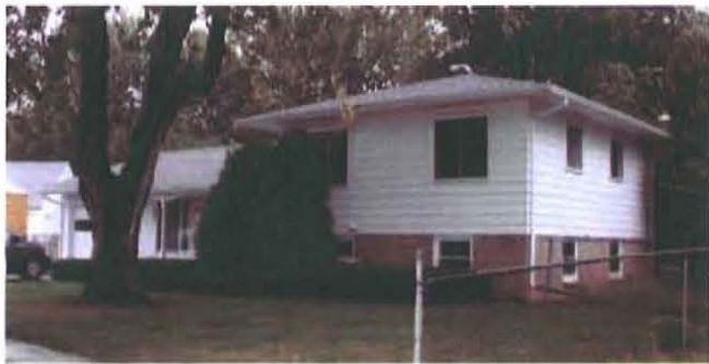
Figure 1. A prefabricated Harnischfeger residence erected c.1960 in the Northbrook Farms Subdivision in Mason, Michigan (Mead & Hunt photograph).
