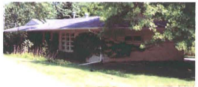
Figure 101. Grouping of 12 Flexivent windows on the rear elevation of a c.1953 Ranch home in Lincoln, Nebraska (Mead & Hunt photograph).
