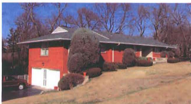
Figure 133. Raised Ranch house in Richmond Heights, Missouri, with the exposed basement at the side elevation, accent stone veneer, and planters (photograph courtesy of Toni Prawl, Missouri Department of Transportation).
