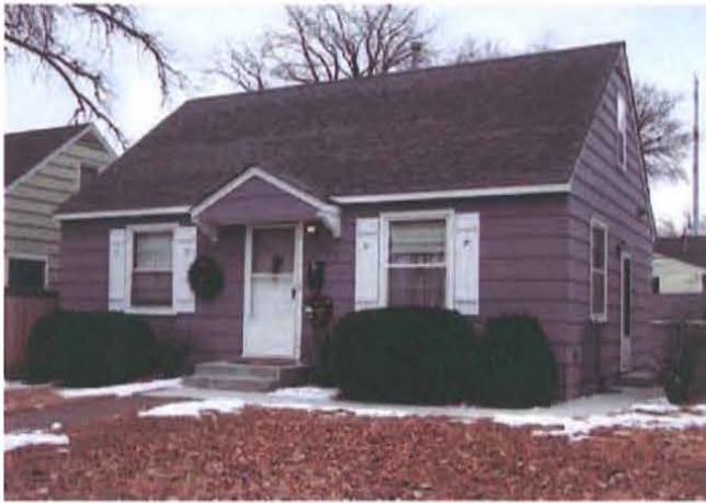
Figure 3. Intact c.1945 house in the postwar St. Louis Park, Minnesota, neighborhood. This residence represents the Minimal Traditional form with a side gable roof. The house retains the original footprint, wide-lap wood siding, and double-hung windows (Mead & Hunt photograph).
