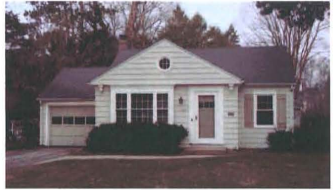
Figure 104. Minimal Traditional house in Madison, Wisconsin, constructed c.1945, with Colonial Revival details, including the decorative pendants and compass window (Mead & Hunt photograph).
