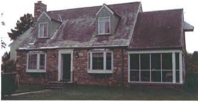
Figure 115. Cape Cod house in Arlington County, Virginia, constructed c.1950, with one-and-one-half-story massing, side gable roof with twin dormers, stone veneer, and sun porch (Mead & Hunt photograph).
