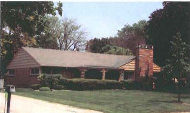
Figure 127. Ranch house in Milwaukee, Wisconsin, constructed c.1960, with horizontal massing, gable roof, stone veneer, accent wood shingles, picture and ribbon windows, prominent chimney, and wrought iron supports at the entrance (Mead & Hunt photograph).
