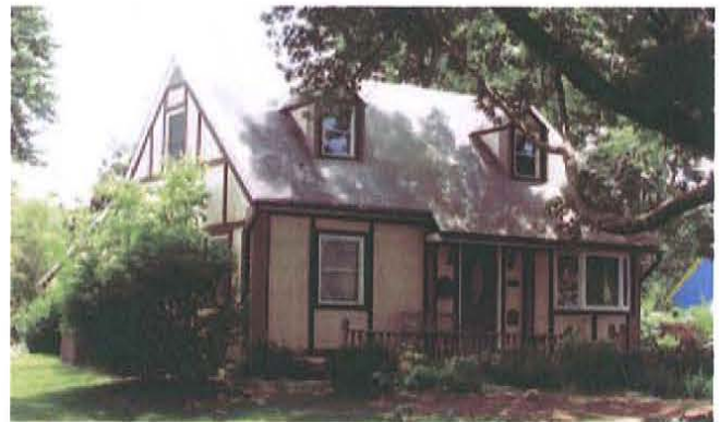
Figure 12. Cape Cod house in Fairfax County, Virginia, constructed c.1945, with exterior cladding altered to create a Tudor Revival appearance, replacement windows and door, and altered stoop. As a result, it does not meet the survey criteria (photograph courtesy of Anne Bruder, Maryland State Highway Administration).
