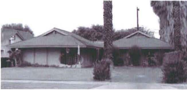
Figure 34. Asiatic residence in Fullerton, California, constructed c.1963, retains its massing and materials and displays architectural elements of the style, including upturned vertical wood trim on the facade and latticework. As a result, it meets the survey criteria (photograph courtesy of Andrew Hope, Caltrans).
