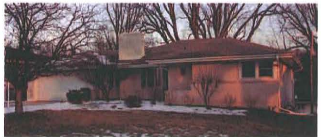
Figure 15. Ranch house in Omaha, Nebraska, constructed c. 1955, retains multiple architectural elements, including accent brick veneer, prominent wide chimney, integrated planter, and wrought iron support, and thus meets the survey criteria (Mead & Hunt photograph).
