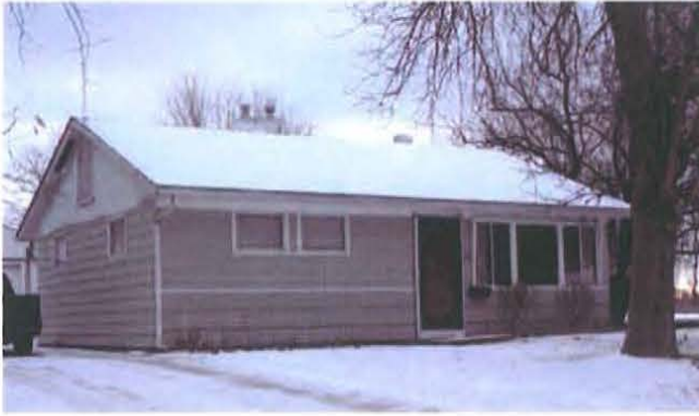
Figure 7. Gunnison house in the Maenner South Addition in Omaha, Nebraska. As one of the most intact of the similar prefabricated c.1955 homes in this addition, it serves as a representative example for the survey documentation (Mead & Hunt photograph).
