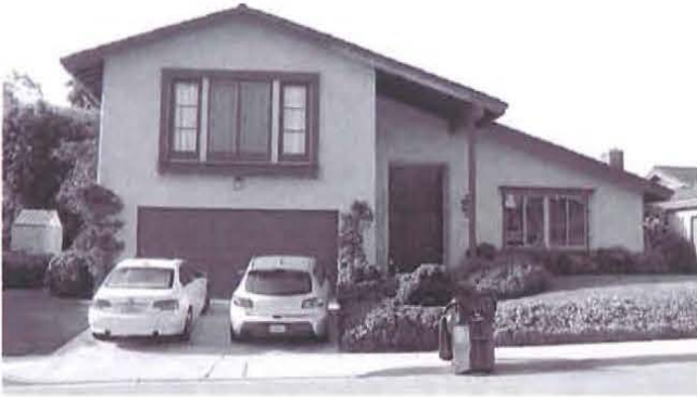
Figure 136. Split-level house in San Diego, California, constructed c.1968, with clearly zoned wings on different levels opening off the centrally located entry, casement windows, and an integrated garage (photograph courtesy of Andrew Hope, Caltrans).
