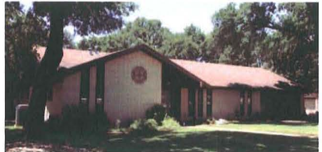
Figure 36. Contemporary house in Arlington, Texas, constructed in 1967, retains its original massing and displays three architectural elements: bands of vertical windows, wrought iron ornamentation on the facade, and Spanish Eclectic stylistic influences. As a result, it meets the survey criteria (Mead & Hunt photograph).
