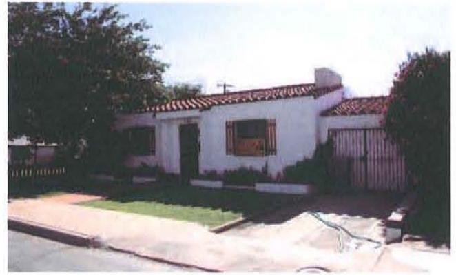
Figure 149. Spanish Colonial Revival style applied to the Ranch form in El Paso, Texas. Constructed c.1950, this house features true adobe construction, red tile roof, and decorative wrought iron details (Mead & Hunt photograph).
