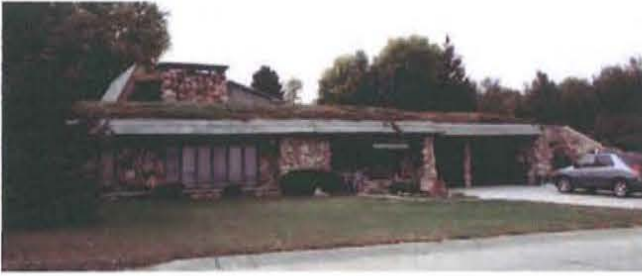
Figure 160. Earthen house in Broken Bow, Nebraska, constructed c.1975 into an embankment with only one exposed elevation (Mead & Hunt photograph).
