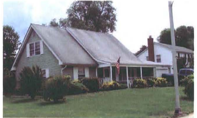
Figure 118. Cape Cod house in Prince George's County, Maryland, with one-and-one-half-story massing, side gable roof, and double-hung windows. The house was constructed by Levitt and Sons in the Belair Subdivision in the early 1960s (photograph courtesy of Anne Bruder, Maryland State Highway Administration).
