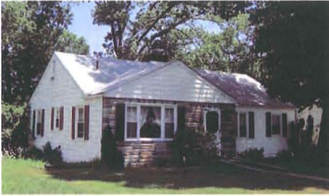
Figure 9. This house in Virginia Heights, built in 1950, is clad with Formstone, a non-traditional material introduced on Arlington houses in the 1950s (Mead & Hunt photograph).
