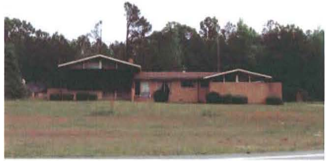
Figure 75. Postwar house in a rural southeast Georgia setting (photograph courtesy of Georgia Department of Natural Resources, Historic Preservation Division).
