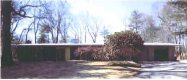
Figure 92. ALCOA Care-free House in Lincoln, Massachusetts, with a white anodized standing seam roof, purple anodized corrugated wall panels, and anodized yellow door cladding (photograph courtesy of John A. Burns, FAIA).
