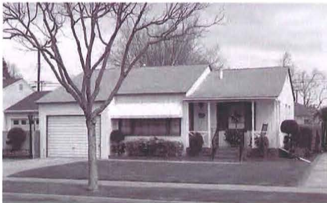
Figure 114. Minimal Traditional house in Lakewood, California, constructed c.1950, with side gable roof, stucco and vertical wood siding, inset entrance, minimal eave overhang, and attached one-car garage (photograph courtesy of Andrew Hope, Caltrans).
