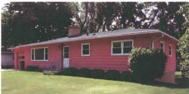
Figure 17. Ranch house in Madison, Wisconsin, constructed in 1958, retains its original massing, siding, and window configuration but does not display three architectural elements and does not meet the survey criteria (Mead & Hunt photograph).
