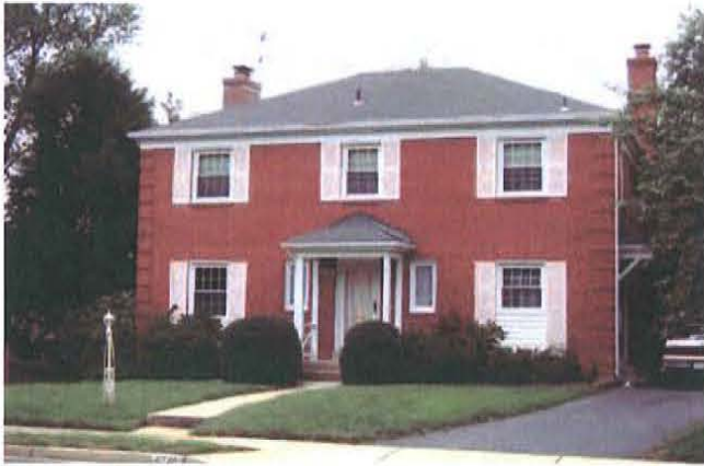
Figure 145. Georgian Revival house in Arlington County, Virginia, with symmetrical front facade, portico, and brick quoins (Mead & Hunt photograph).
