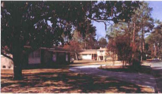
Figure 43. Ranch and Split-level house in the Fairway Oaks-Greenview Historic District in Savannah, Georgia (photograph courtesy of Georgia Department of Natural Resources, Historic Preservation Division).
