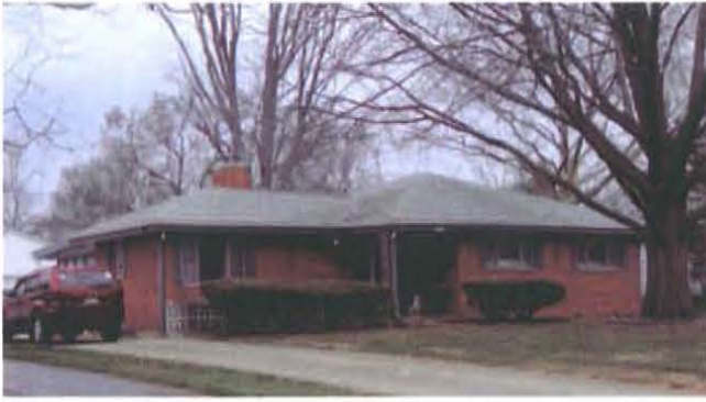
Figure 103. Ranch house in Upper Arlington, Ohio, constructed c.1955, with a hip roof, brick veneer, recessed entrance with decorative wrought iron details, and decorative shutters (Mead & Hunt photograph).
