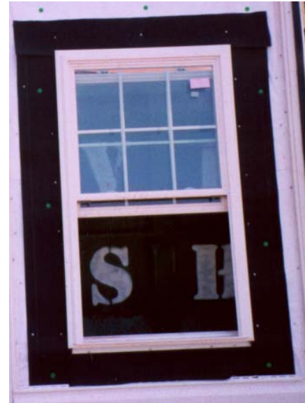
Figure 3 Flashing Detail
