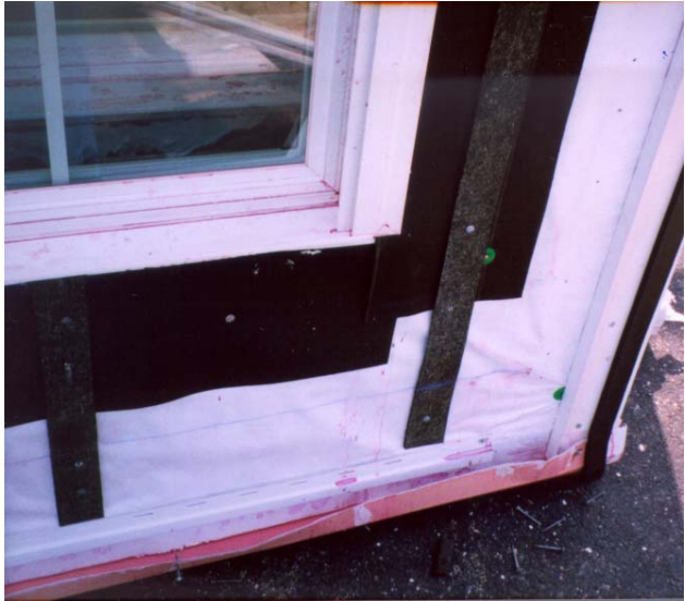
Figure 13 Fiber Cement with Drainage Plane (Window)
