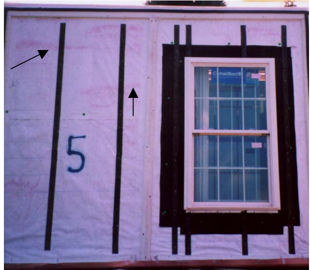
Figure 14 Fiber Cement with Drainage Plane
