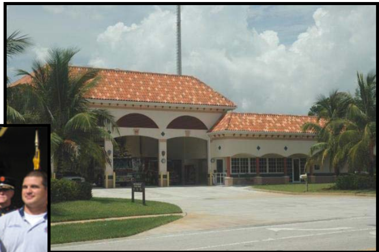
Firehouse No. 57 opened in 2002 and serves as the 5 th Battalion Headquarters.
