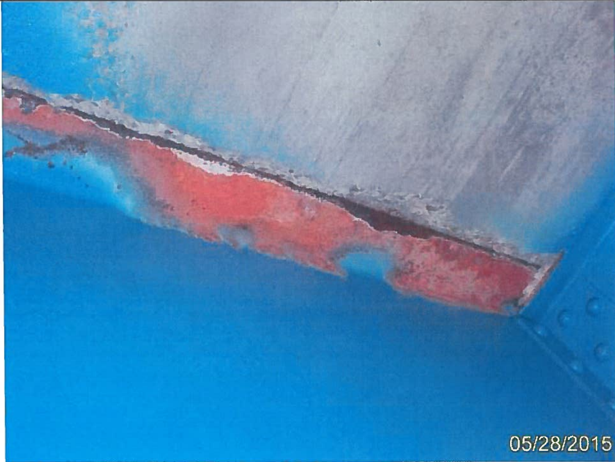
Photo 58 – Unit 1 Element 152 Paint Stl Floor Beam
