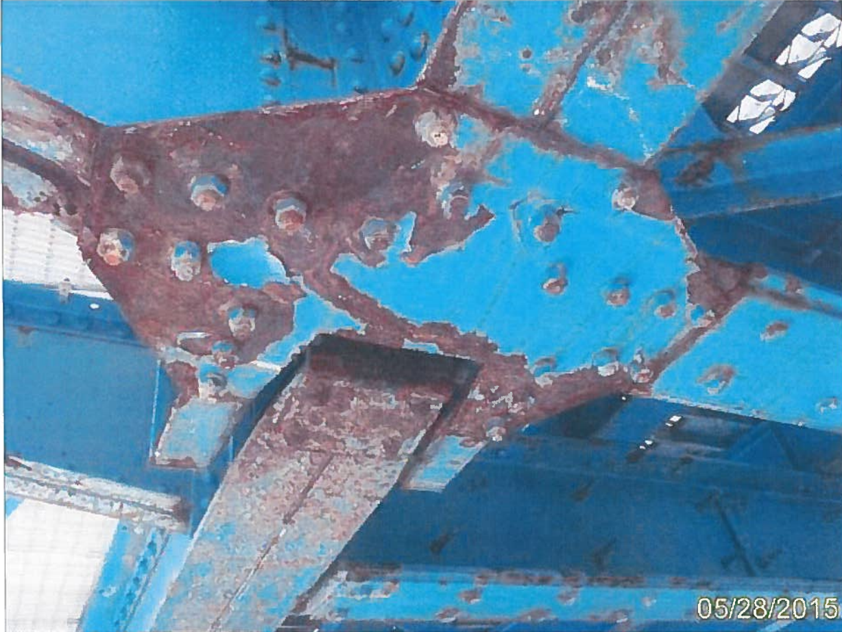
Photo 9 – Unit 0 Element 152 Paint Stl Floor Beam
