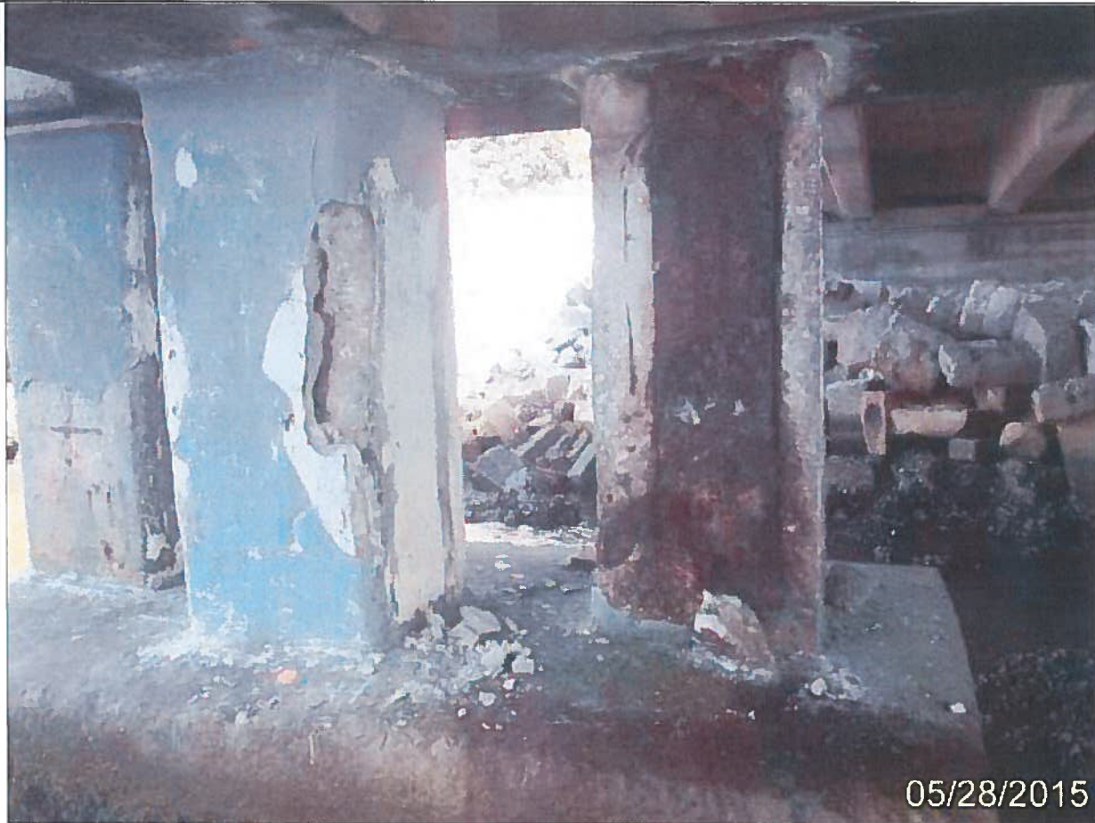
Photo 60 – Unit 1 Element 202 Paint Stl Column
