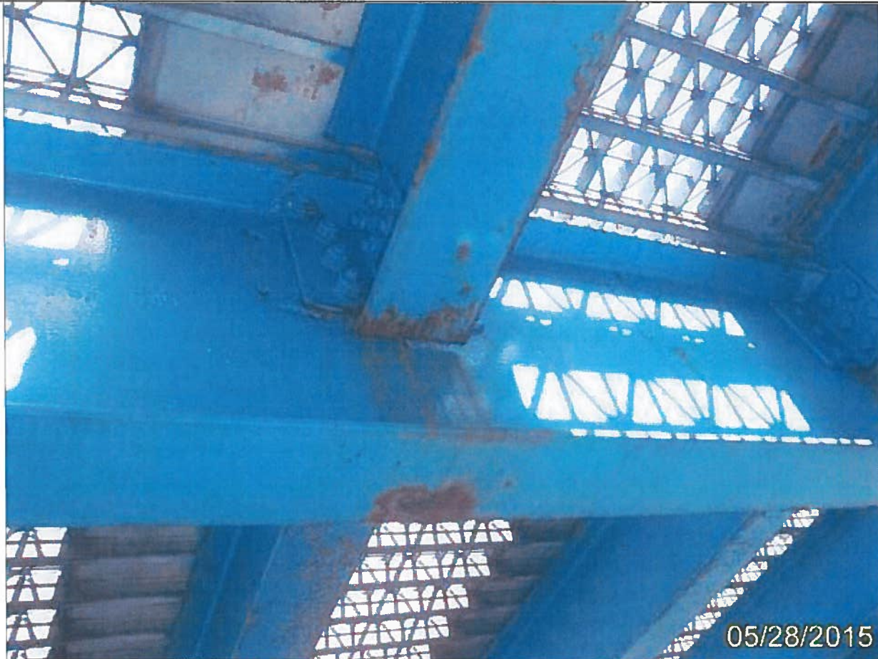
Photo 6 – Unit 0 Element 113 Paint Stl Stringer
