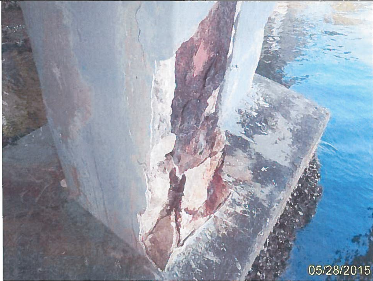
Photo 61 – Unit 1 Element 202 Paint Stl Column
