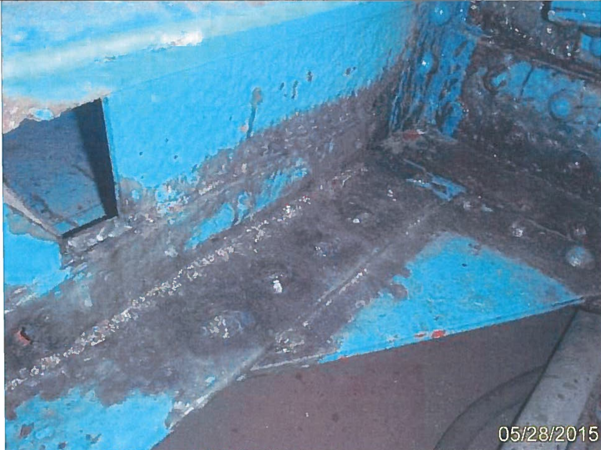
Photo 5 - Unit 0 Element 107 Paint Stl Open Girder
