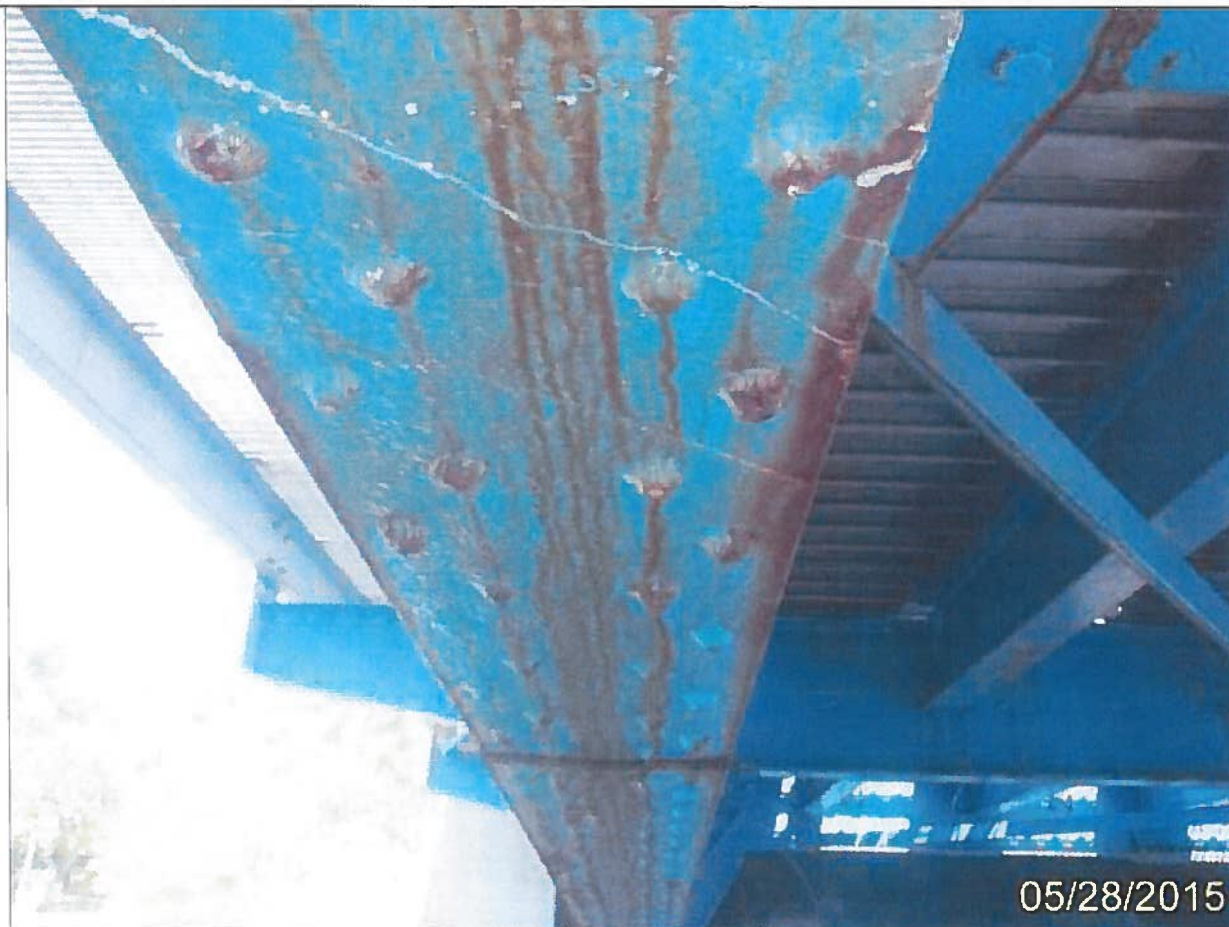
Photo 3 – Unit 0 Element 107 Paint Stl Open Girder
