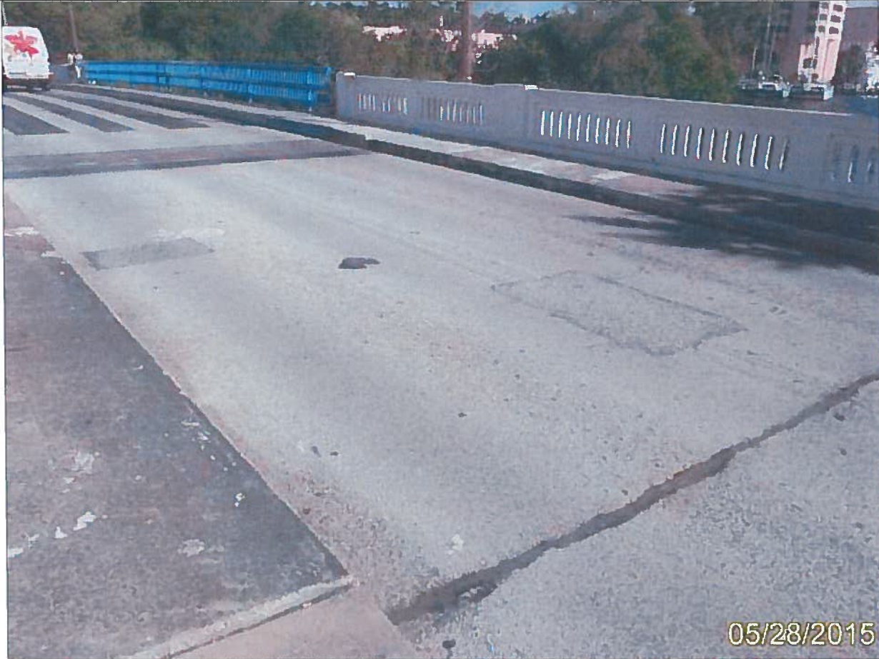
Photo 48 – Unit 1 Element 13 Unp Conc Deck/Asp Ovl
