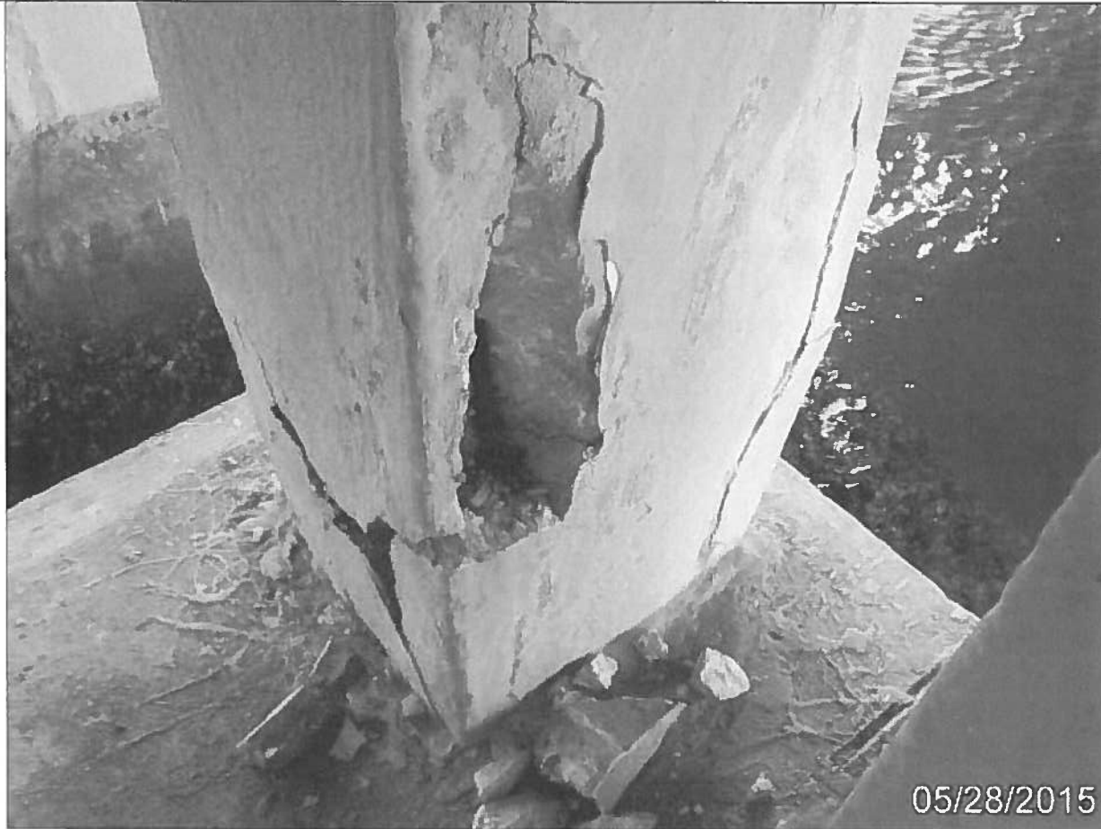
Photo 63 – Unit 1 Element 298 Pile Jacket Bare
