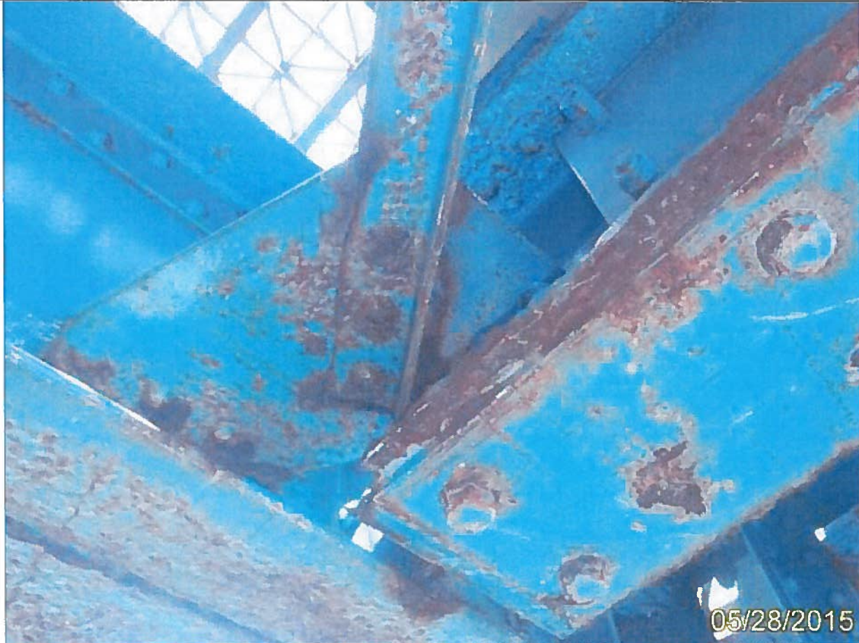
Photo 10 – Unit 0 Element 152 Paint Stl Floor Beam
