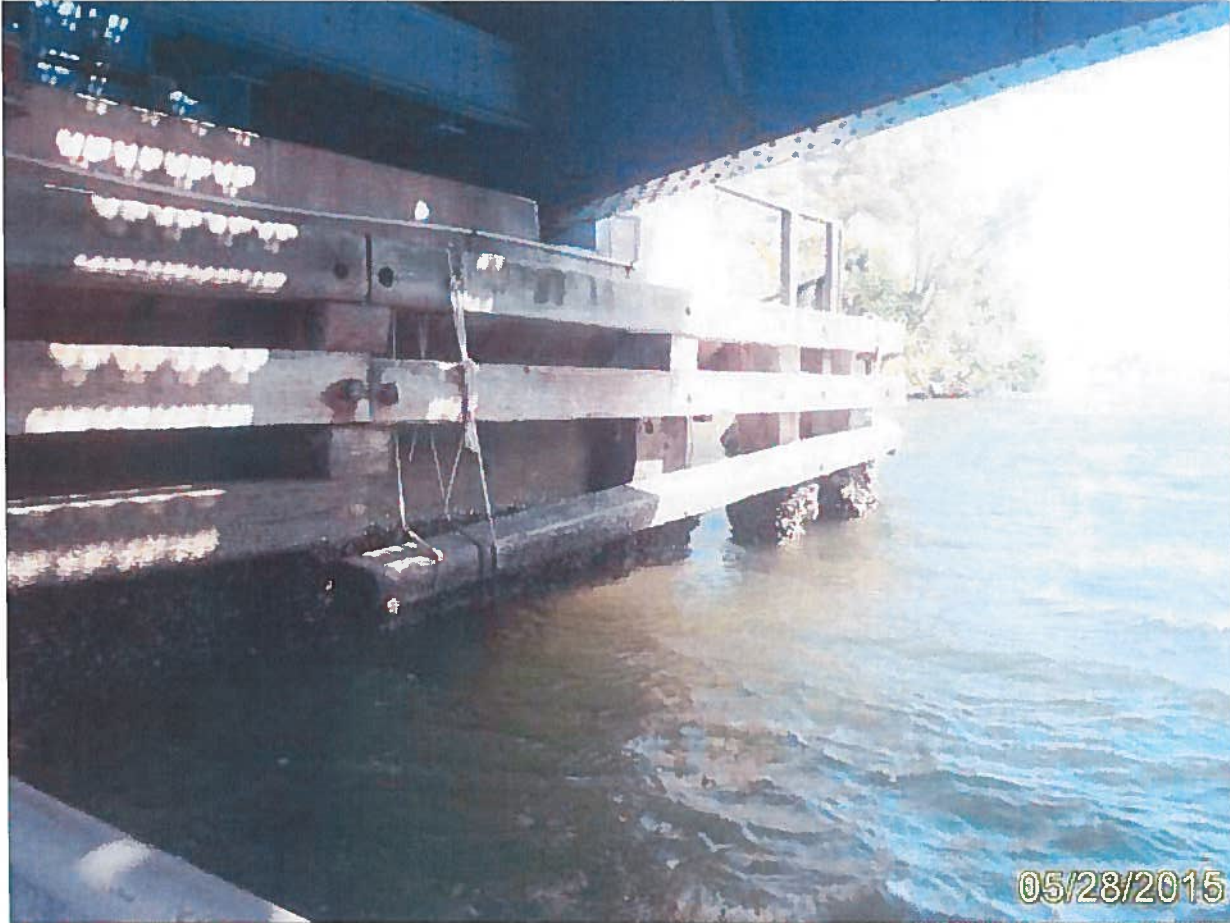
Photo 66 – Unit 1 Element 387 P/S Fender/Dolphin
