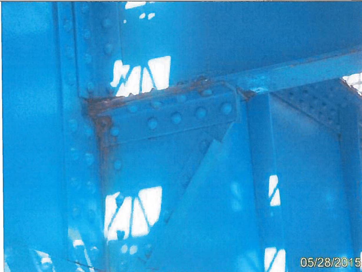
Photo 8 – Unit 0 Element 152 Paint Stl Floor Beam
