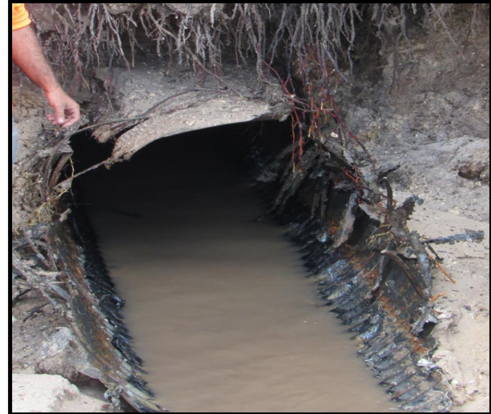
Corroded CMP sinkhole
