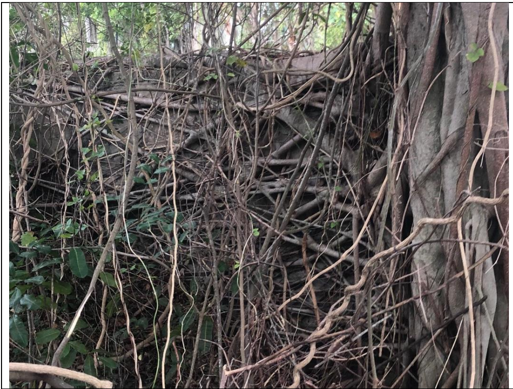
Figure 44 Interior side of northwest wall
