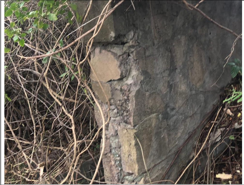
Figure 43 Northwestern CBS wall on High ridge area of County Home
