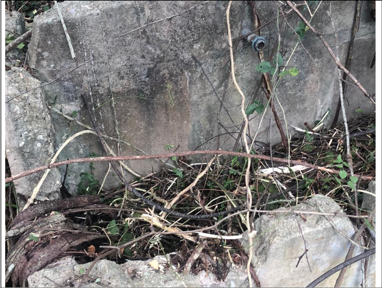
Figure 42 Large cement basin with water line in High Ridge Structure
