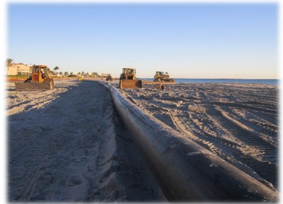
Bull dozers shape sand pumped to the beach via pipeline.
