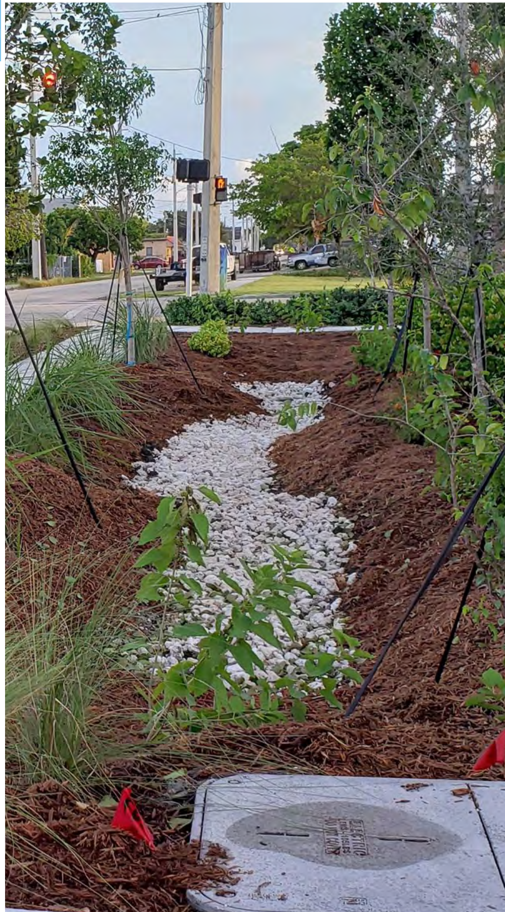
Example of bioswale to treat and retain stormwater (Photo credit: City of Hallandale Beach, FL)
