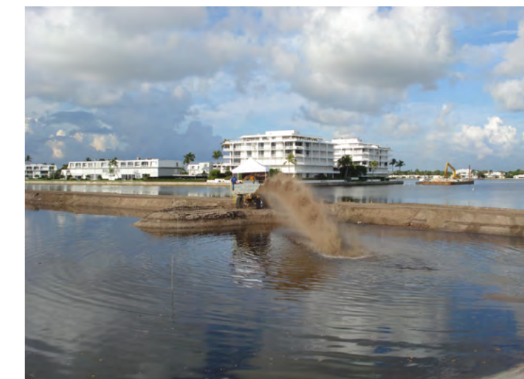
Sand shooter in use at Ibis Isle restoration (Photo credit: PBC-ERM)
