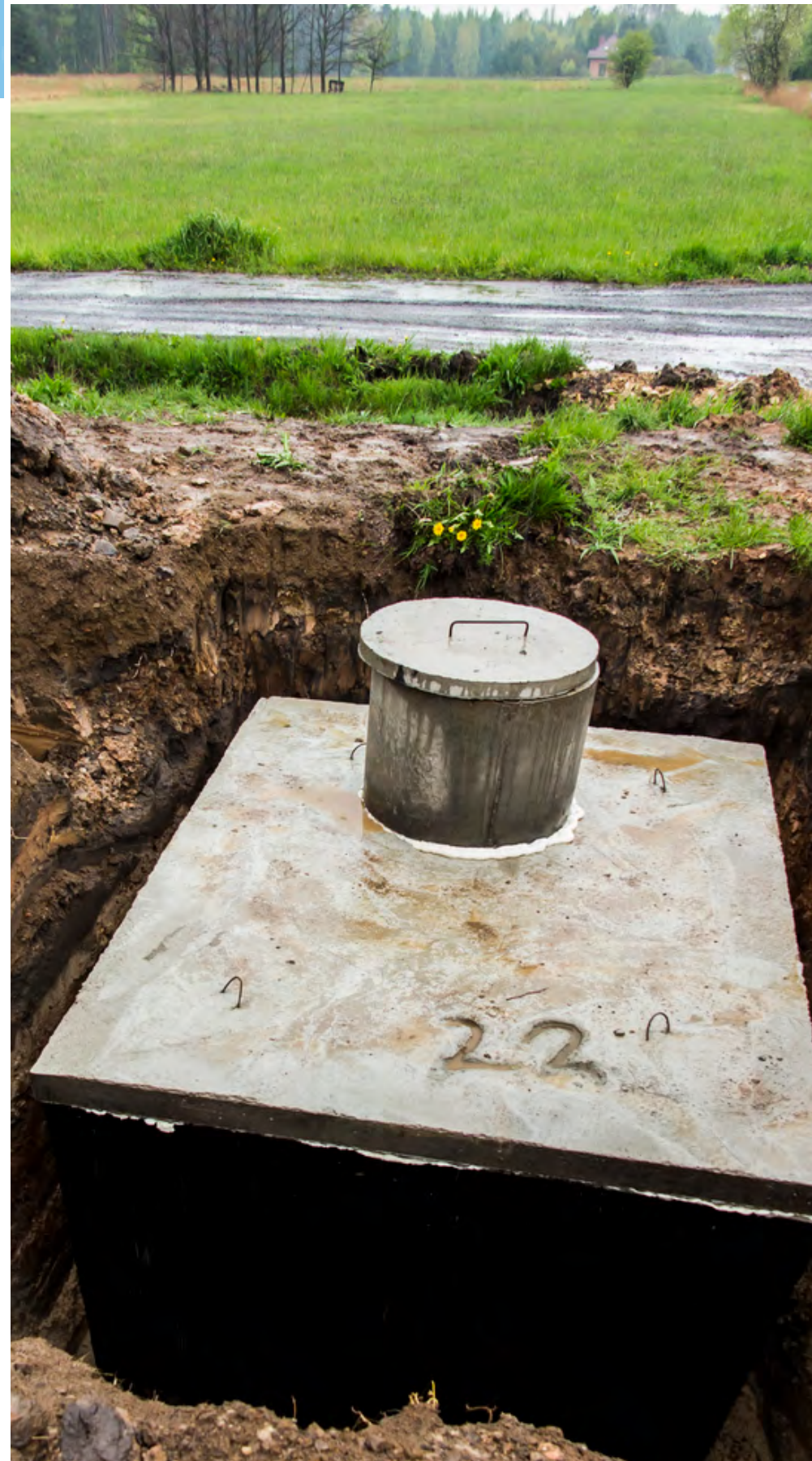
Septic system being installed (Photo credit: Stock photo/Dreamstime)
