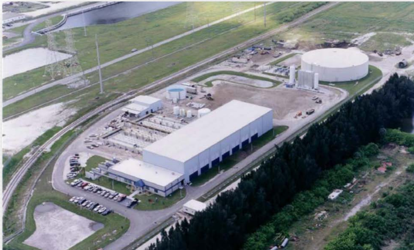
Tampa Bay Water's desalination plant.
