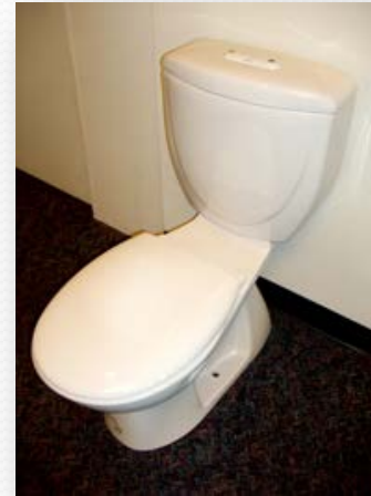
Dual flush toilet: Uses 0.8 to 1.6 gpf
