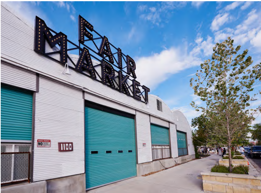
1100 East Fifth St. – Restoration of a 16,000 sq. ft. metal Quonset hut into one of the premiere private events facilities in Austin.
