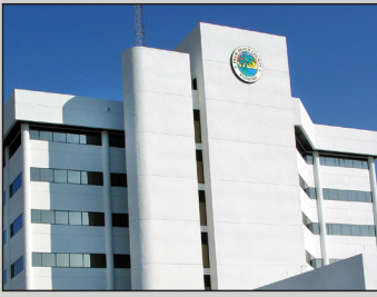
The central administrative office is located at 301 N. Olive Ave., West Palm Beach.
