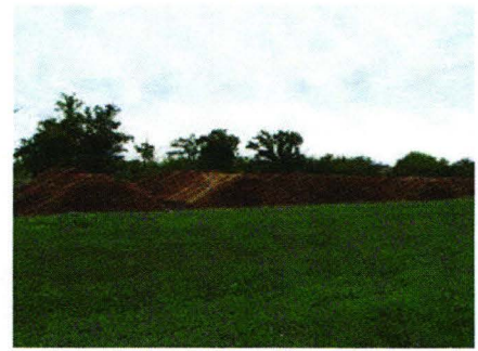
Figure 3. Compacted clay composting pad
