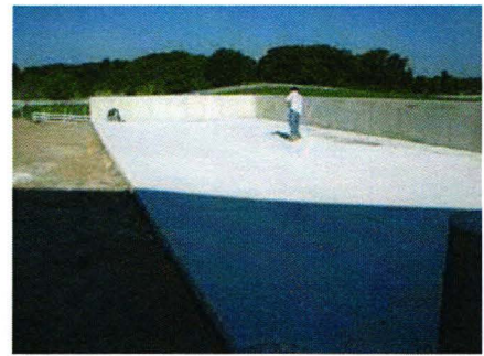
Figure 2. Concrete manure storage pad
