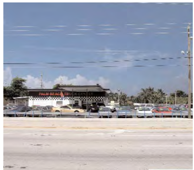
Much of the development on Military Trail is low-scale, out-dated commercial structures many of which are auto-oriented
