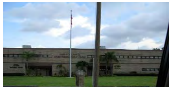
The PBLA industrial site is adjacent to the Armed Forces Reserve Center on Gun Club Road
