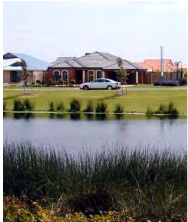
Wet detention pond
