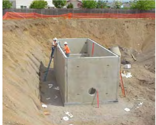
Underground storm water vault
