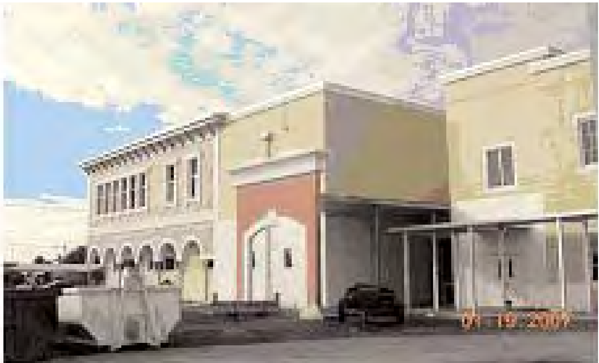
The Berkshire Elementary School in the City of West Palm Beach is undergoing substantial expansion and renovation
