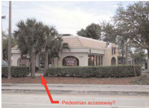
Pedestrian access from the sidewalk to the restaurant, which is adjacent to a bus stop, is not defined
