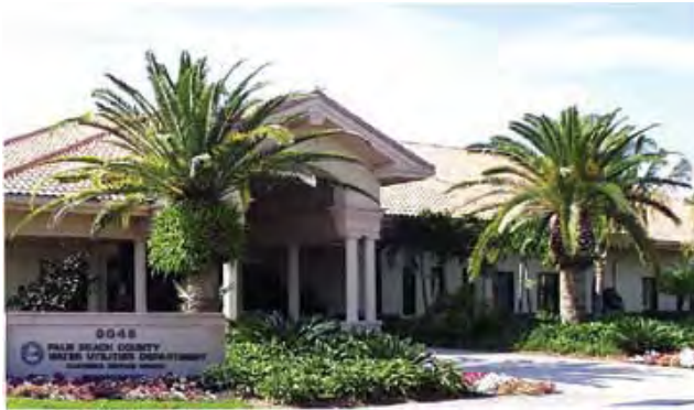
The Palm Beach County Water Utilities Department
