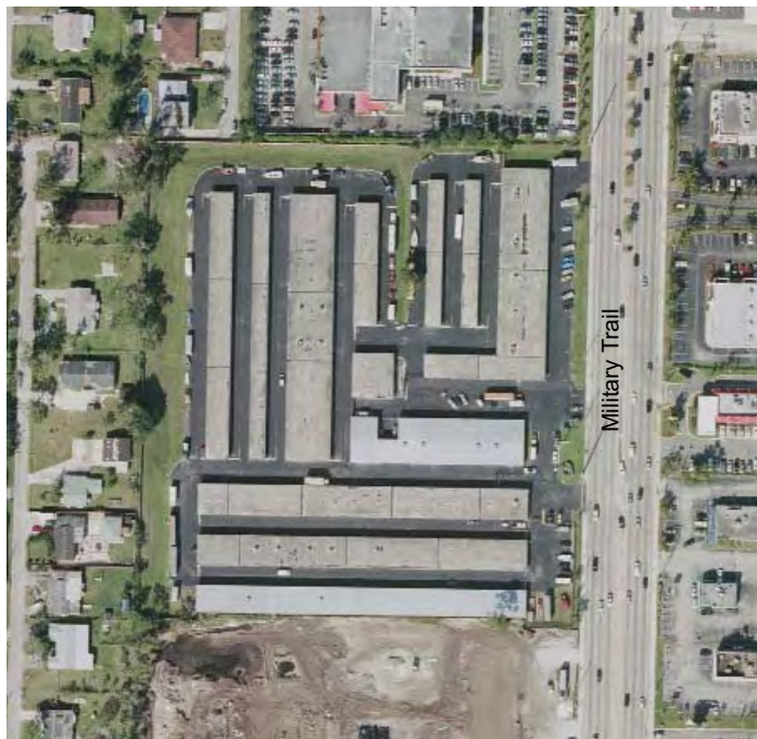
The existing storage facility is a series of one-story, non-descript buildings that cover the entire site.
