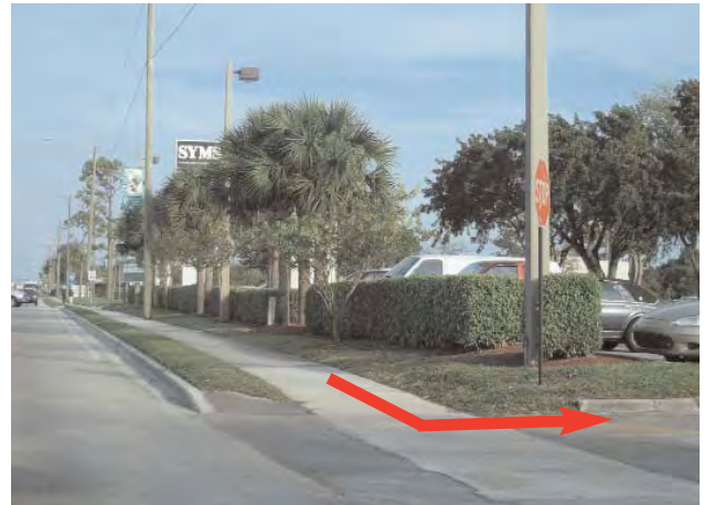
In the absence of a defined pedestrian path, the driveway is used for access increasing the potential for vehicular/ pedestrian conflicts
