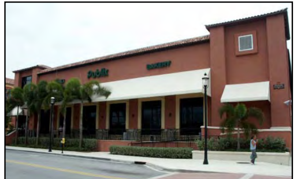
The Publix at CityPlace shows how a grocery store can fit successfully into an urban environment: the building addresses the street, and the parking is shielded from the street
