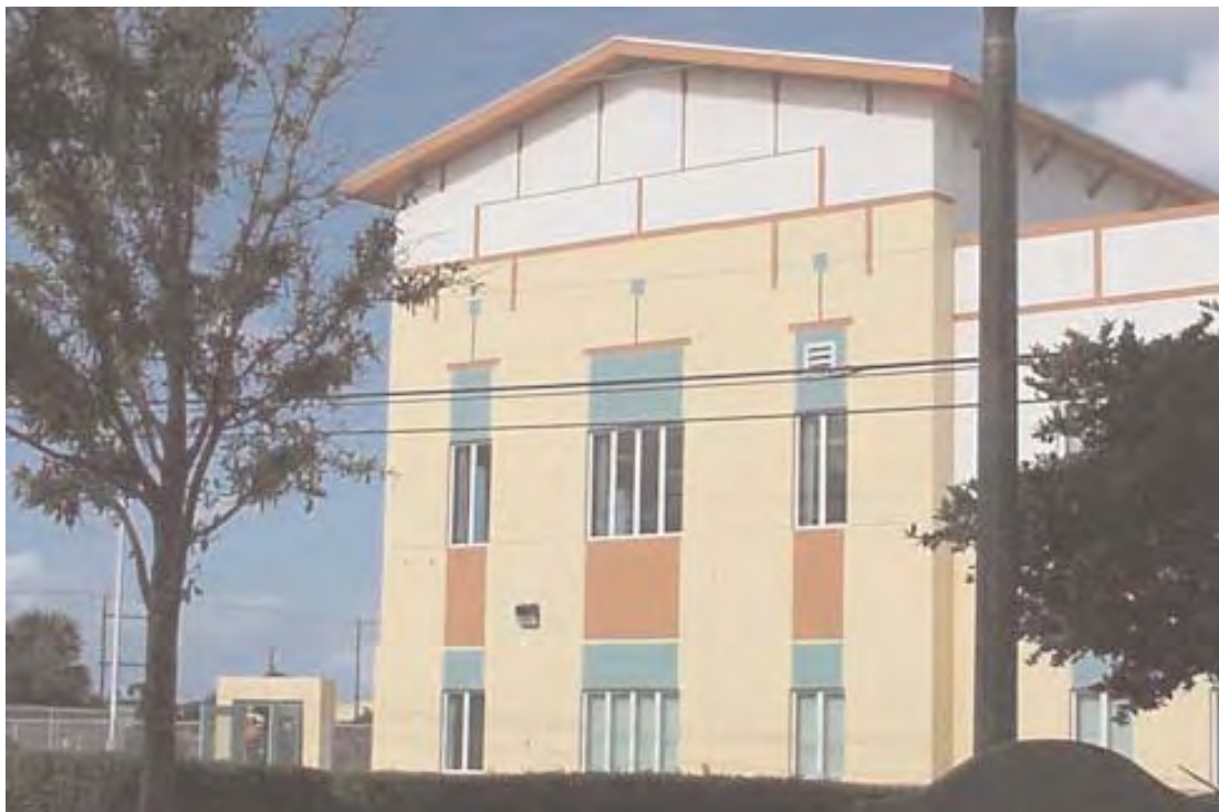
Pleasant City Elementary School in the City of West Palm Beach, which opened in 2002, was the first new urban school built by the district in decades
