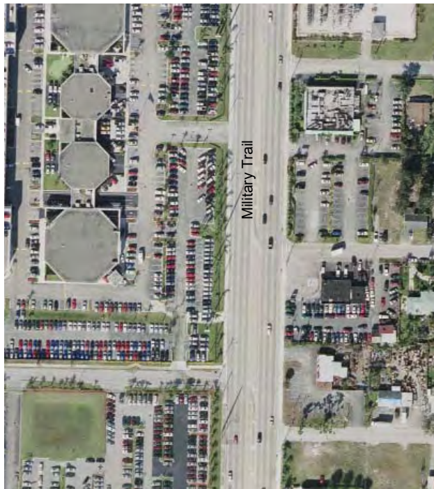
In the current condition, it is virtually impossible to travel from one adjacent parcel to another without going onto Military Trail
