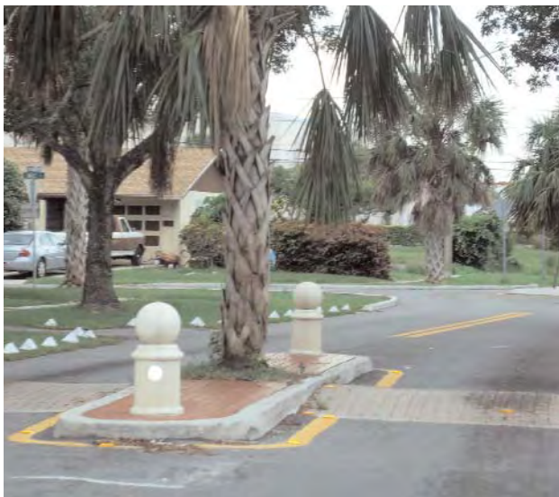
Some neighborhoods within the URA have an established traffic calming program with interventions, like this one above, that not only slow local traffic but also serve as beautification elements.
