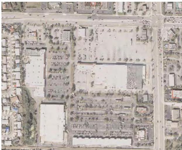
Aerial view showing the existing conditions of the Sears plaza at Military Trail and Forest Hill Boulevard
