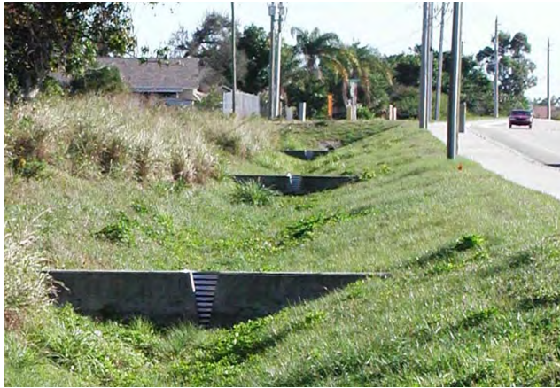
Large swale with "V"-notch weir designed to provide both conveyance and detention of storm water
