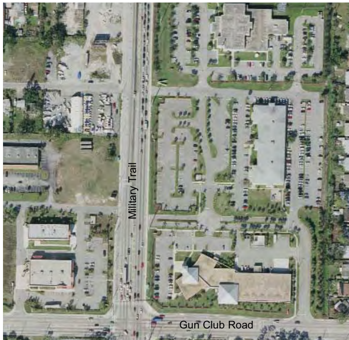
The current situation: berms and parking lots define Military Trail making it a lonely and dangerous place to be a pedestrian
