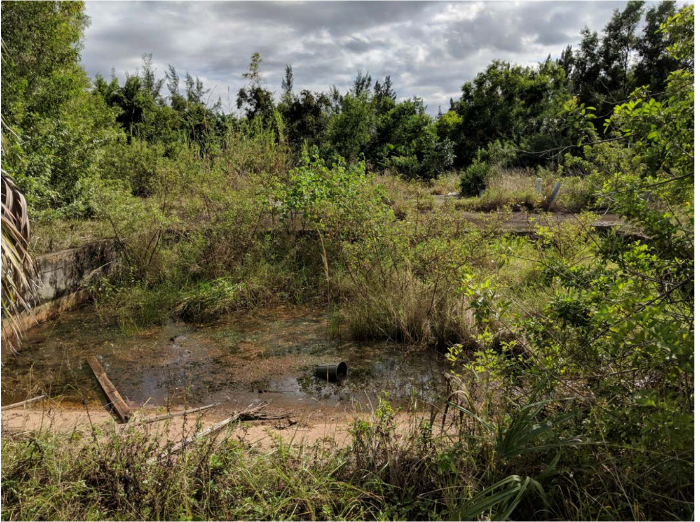
Photo 2. This photo, facing south, shows the loading bay in the portion of the subject property that had been used as a field nursery. Behind the concrete incline used as a truck bay, there used to be a building. Although there is standing water on the concrete incline, this area was not identified as an Other Surface Water due to the concrete flooring.
