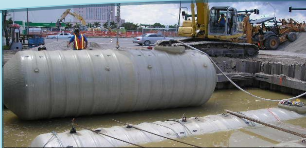
Underground storage tank systems are often installed in high ground water levels in Palm Beach County
