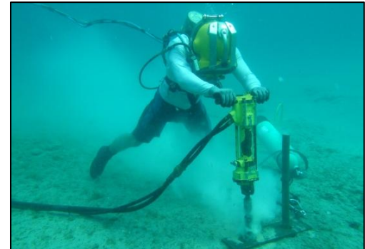
Anchor pin installation
