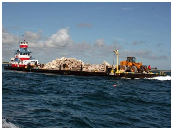
Concrete/limestone rock deployed in 2010
