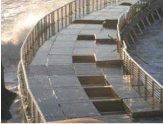
Left: North jetty deck panels displaced and railing damaged during Hurricane Sandy in October 2012.
